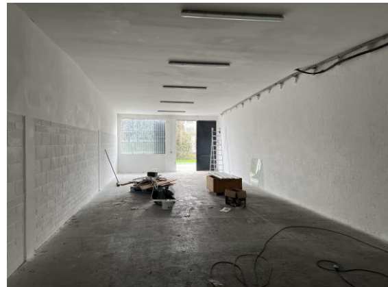
Unit photographed while undergoing refurbishment.
